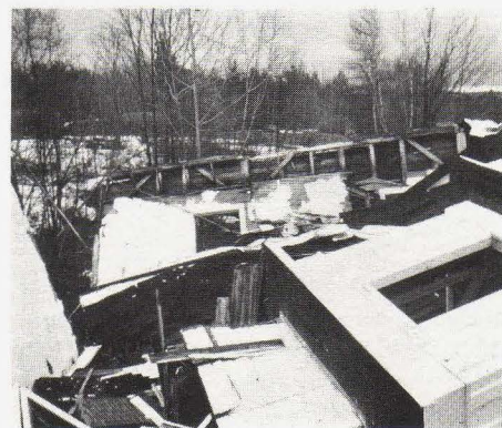
THE CHURCH was destroyed on March 10, 1969 by an excess weight of snow on the roof.
