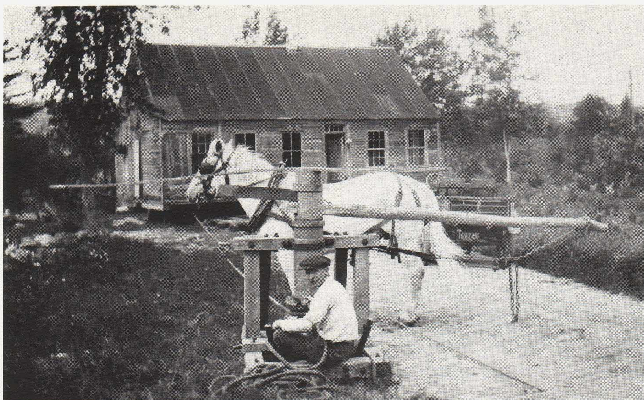
Primitive moving facilities employed to transfer the North Groton house to its original site.
