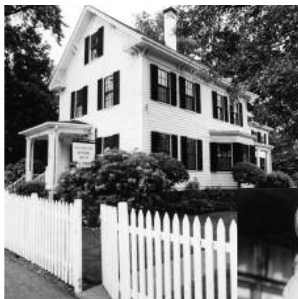
This significant historical landmark in Swampscott will benefit from exterior restoration. Wooden clapboards and trim will be repaired and painted to protect the structure from water, weather and pests.
