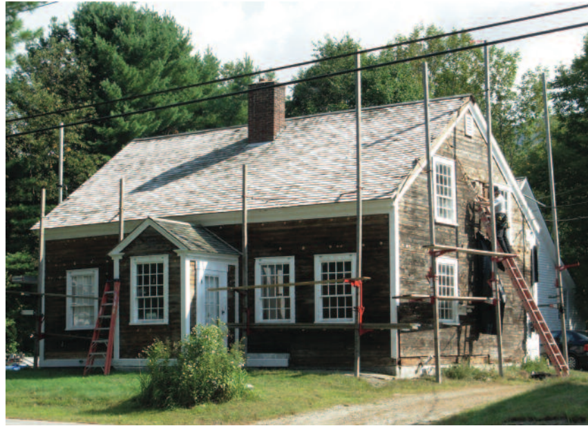
The craftsman (on ladder on right) is investigating the joints where the sheathing for the original saltbox house meets the later addition.
