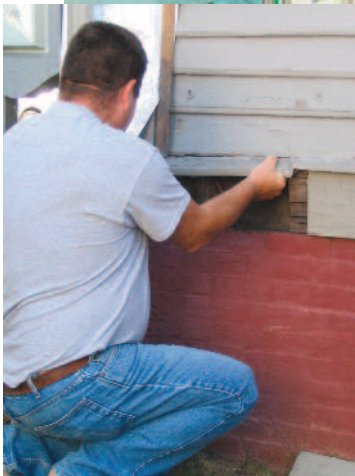
Removing clapboards to find remnants of original paint color.
