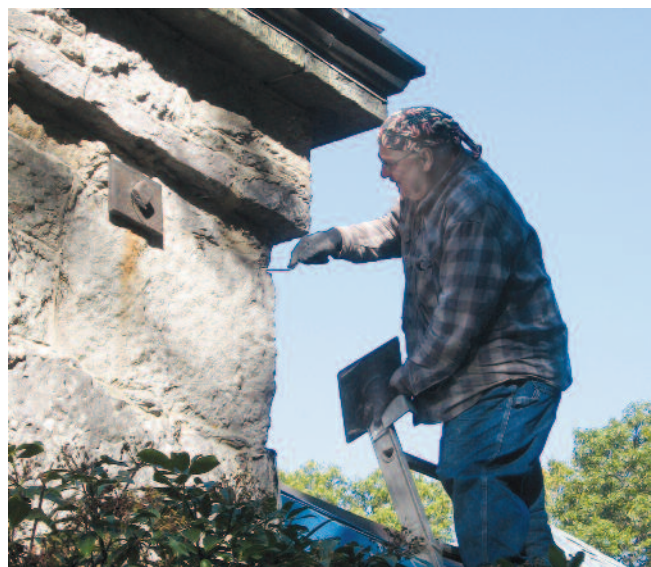
Masons repointed a section of the stone wall, as part of the Chestnut Hill Carriage House roof project last summer.
