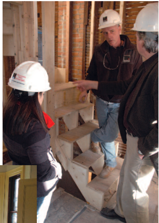
Clockwise from upper left: first floor parlor door being restored to its original location, while stairs in the background will be rotated 90° back to their original location; members of the restoration team discussing the back stairs as they are being rebuilt in their original location; work in progress, first floor parlor; installing new trim, second floor kitchen.
