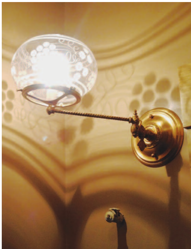
Period gas-light fixture, second-floor pantry. Original gas-pipe opening is visible below the now-electrified fixture.
