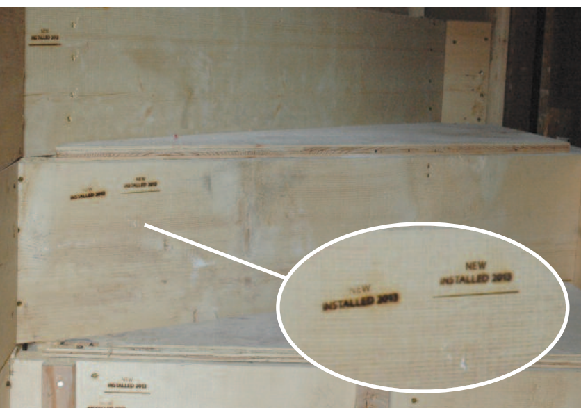
New materials used in reconstruction were marked with date so future investigators would easily recognize work done in 2013.
