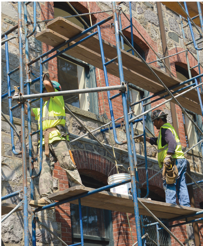
Masons repoint mortar on the south side of 400 Beacon Street's façade.
