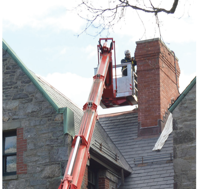
A worker gets a lift in a “cherry picker” to install flue venting and a copper cap on the chimney.
