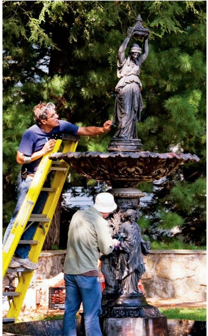
Conservation engineer Jean-Louis Lechevre and an assistant restore the finish on the Pleasant View fountain in 2011.
